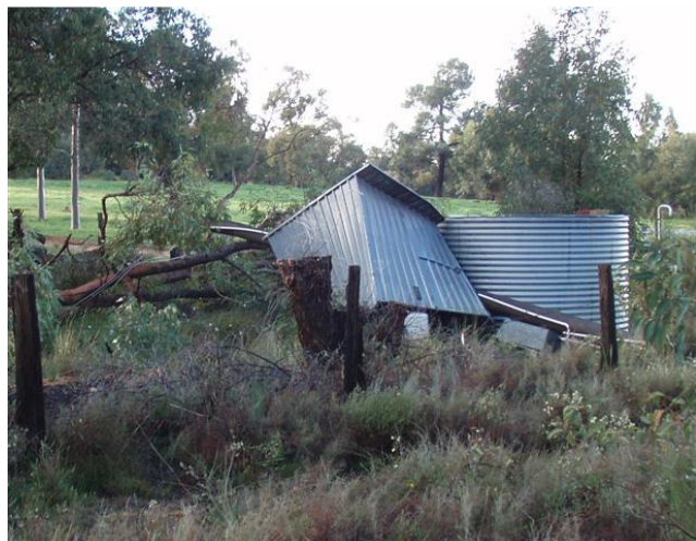
Images showing damage to the water pump station shed. The shed was hit with a tree and a power pole.
