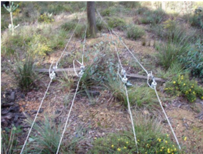
Fallen power lines on site
